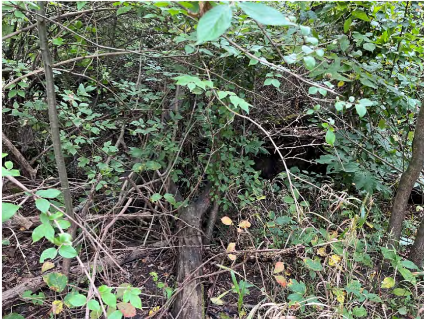
Photo 201. Looking southeast at Erosional Feature 1 which drains Wetland 11-A.
