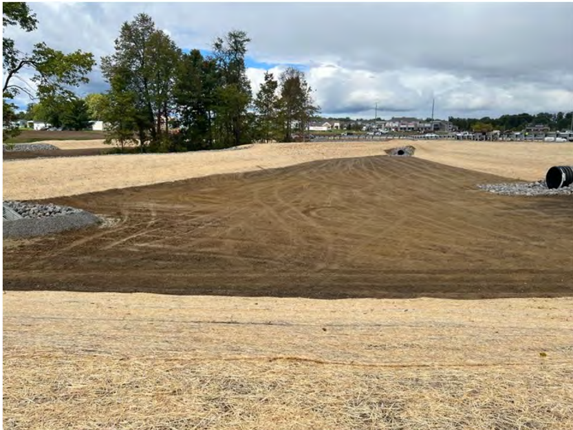
Photo 135. Looking northwest at a dry bottom retention pond currently under construction.
