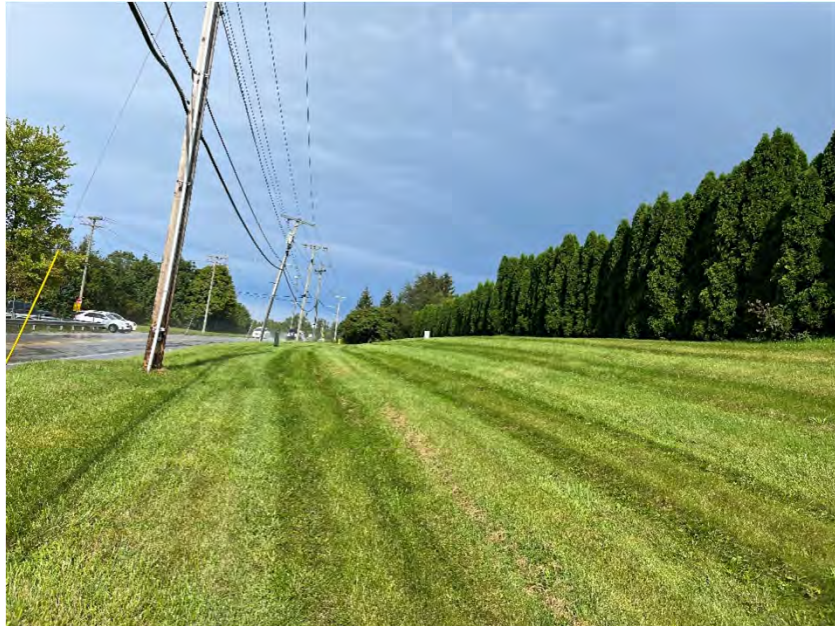
Photo 189. Looking northeast at maintained grassy ROW.
