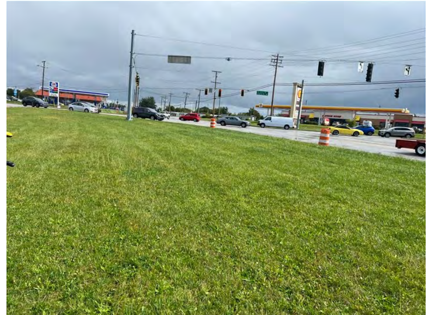
Photo 138. Looking northeast at maintained grassy ROW towards the northern extent of the project area.
