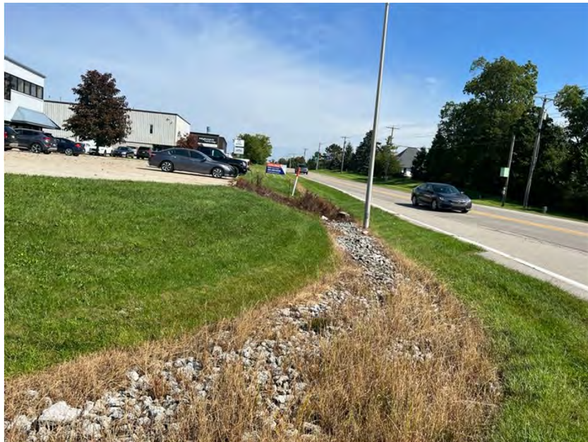
Photo 57. Looking north at a riprap lined roadside ditch.
