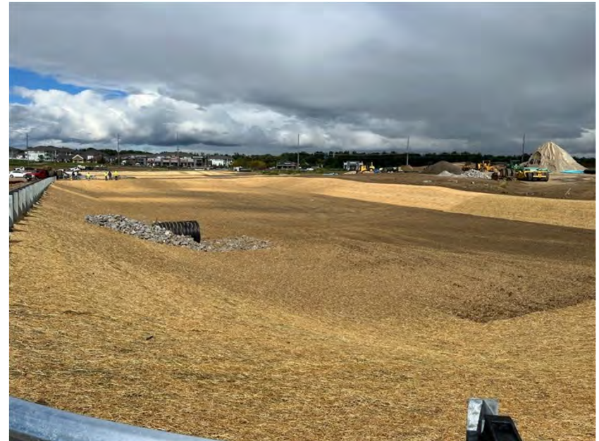
Photo 136. Looking northwest at a dry bottom retention pond currently under construction.
