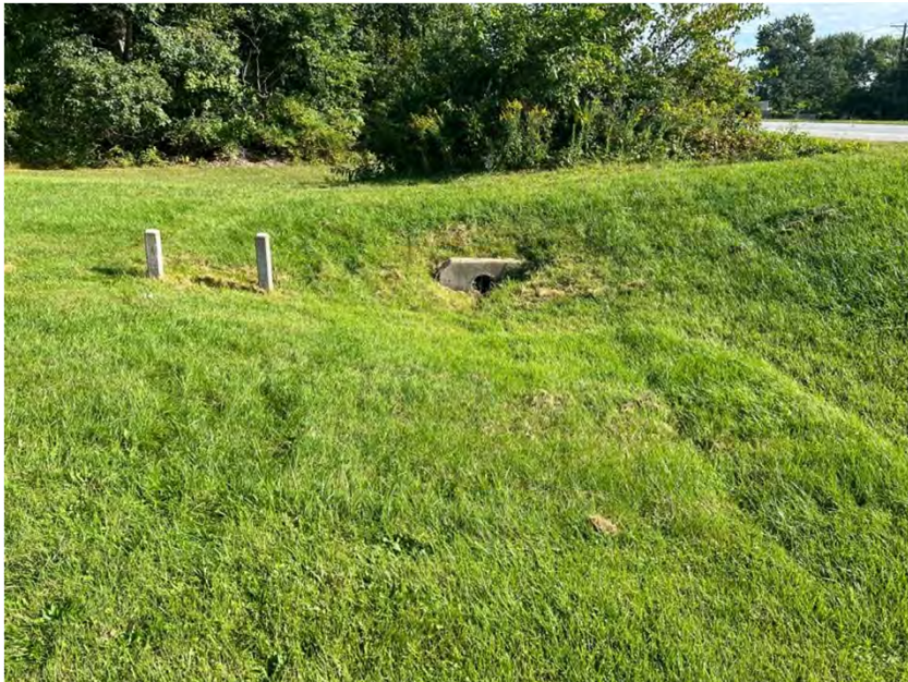
Photo 11. Looking north at culvert outlet and maintained grassy ROW.
