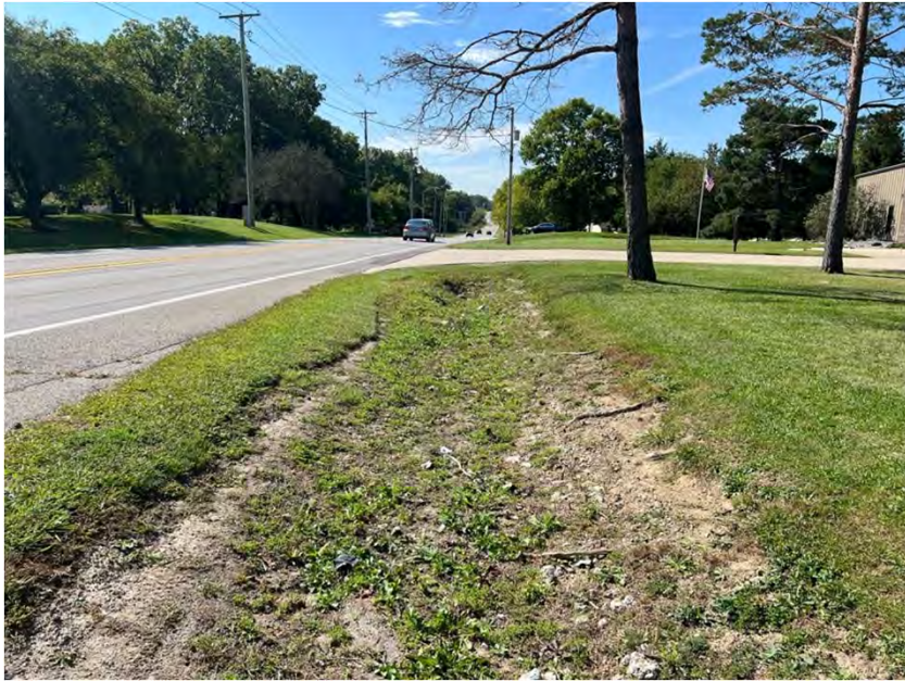
Photo 53. Looking south at a roadside ditch and driveway culvert inlet.
