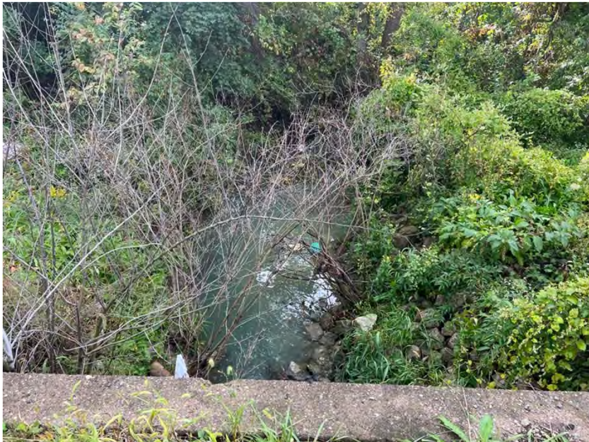
Photo 151. Looking southeast at Martin Ditch.
