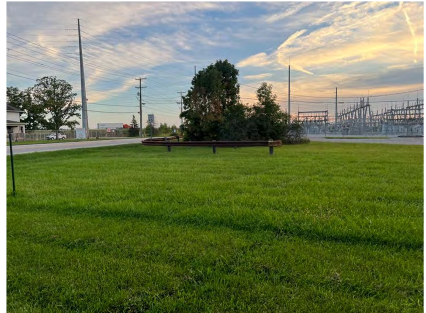
Photo 120. Looking southwest at maintained grassy ROW.
