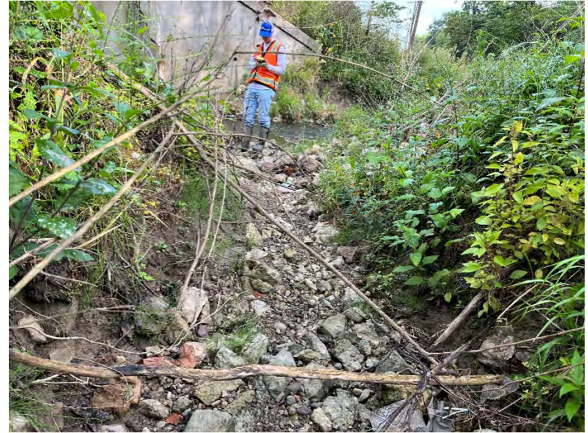
Photo 218. Looking north at a riprap chute which drains into Beckett's Run.
