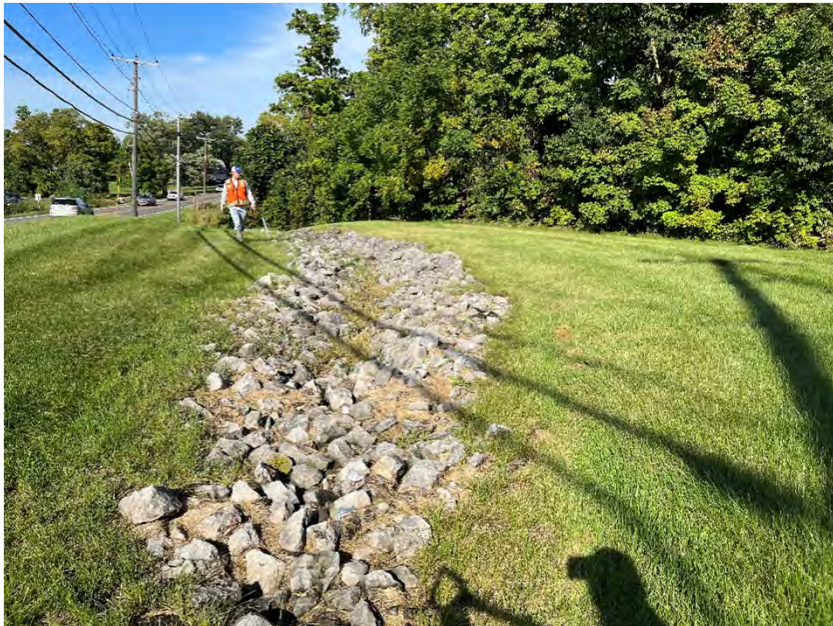
Photo 203. Looking northeast at a riprap chute which drains to Swift Ditch.
