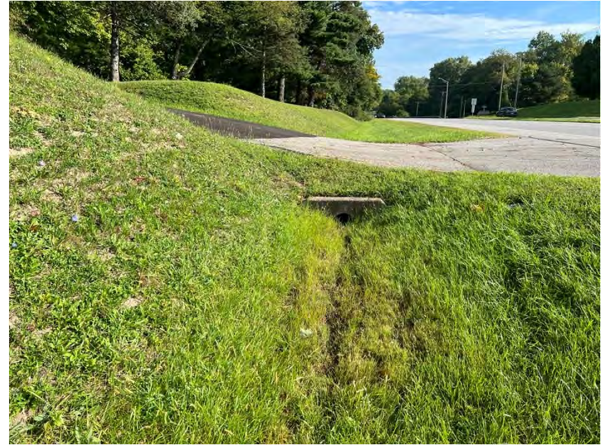
Photo 22. Looking north at culvert outlet and maintained grassy ROW.
