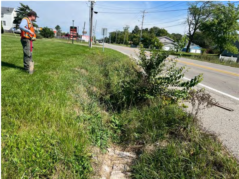
Photo 55. Looking north at a small erosional feature and grassy ROW.
