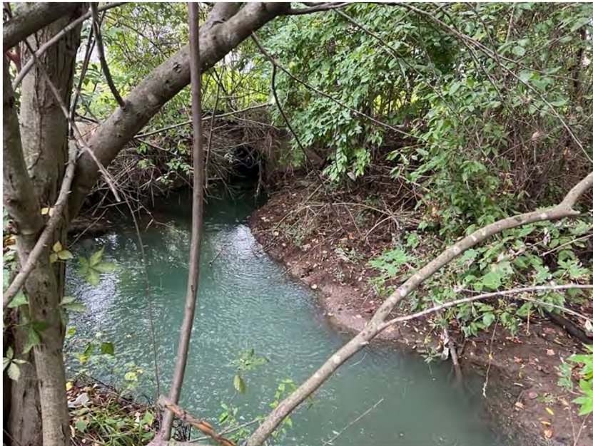
Photo 131. Looking southeast at Martin Ditch and the small structure that conveys the stream under Clinton Street.
