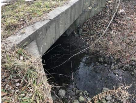
Martin Ditch Structure
