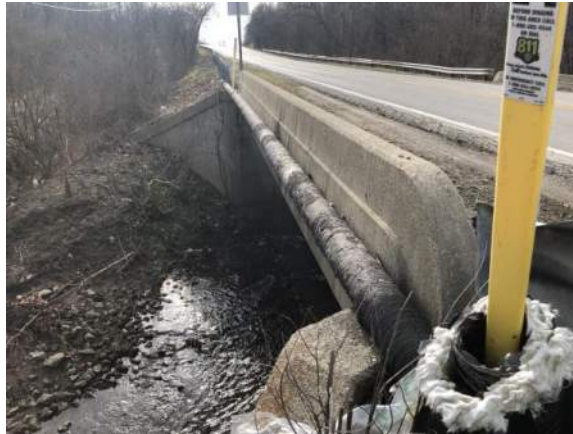
East Side of Becketts Run Bridge Looking South
