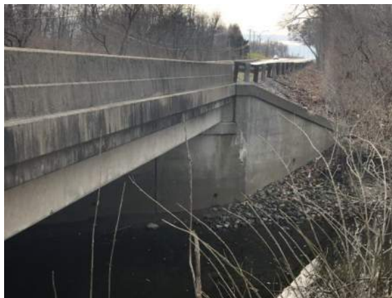
West Side of Becketts Run Bridge Looking South
