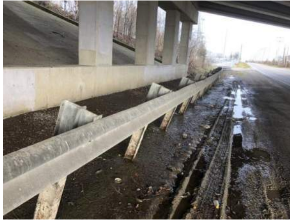
West Side of Clinton Street Looking North Under I-469 Bridge
