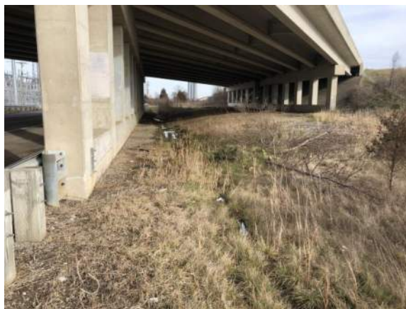
East Side of Clinton Street Looking North Under I-469 Bridge
