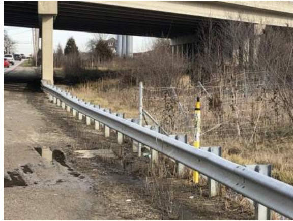
East Side of Clinton Street Looking North Towards I-469 Bridge
