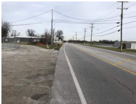
West Side of Clinton Street Looking North Towards Diebold Road
