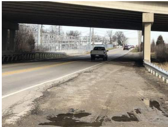
Clinton Street Looking North Towards I-469 Bridge
