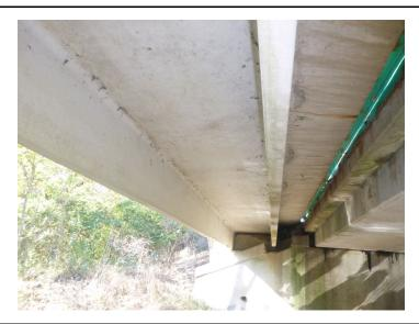
DOUBLE-TEE BEAM FOR SIDEWALK ON SOUTH COPING
